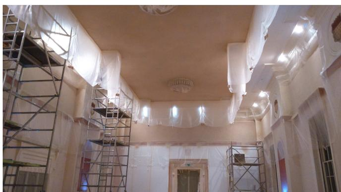
All the lighting is being upgraded with energy efficient LED fittings and the circuitry is being altered to allow more flexibility in lighting mood.
