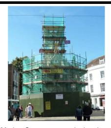
The Market Cross stonework cleaning and restoration works are progressing well and are on schedule. Moss and lichen have been removed and a shelter-coating will be applied to some of the stonework. All the work is being overseen by Historic England.
