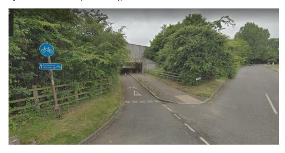
3.1.2 To meet the required headroom, the underpass would have to be lowered which would mean regrading both the approaches. This would be a major engineering exercise, costly and possibly create drainage issues in that the new road level would require pumps operating 24/7 to be installed to prevent flooding.
