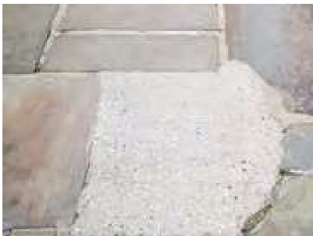
Figure 6.3: Slab infill with concrete
