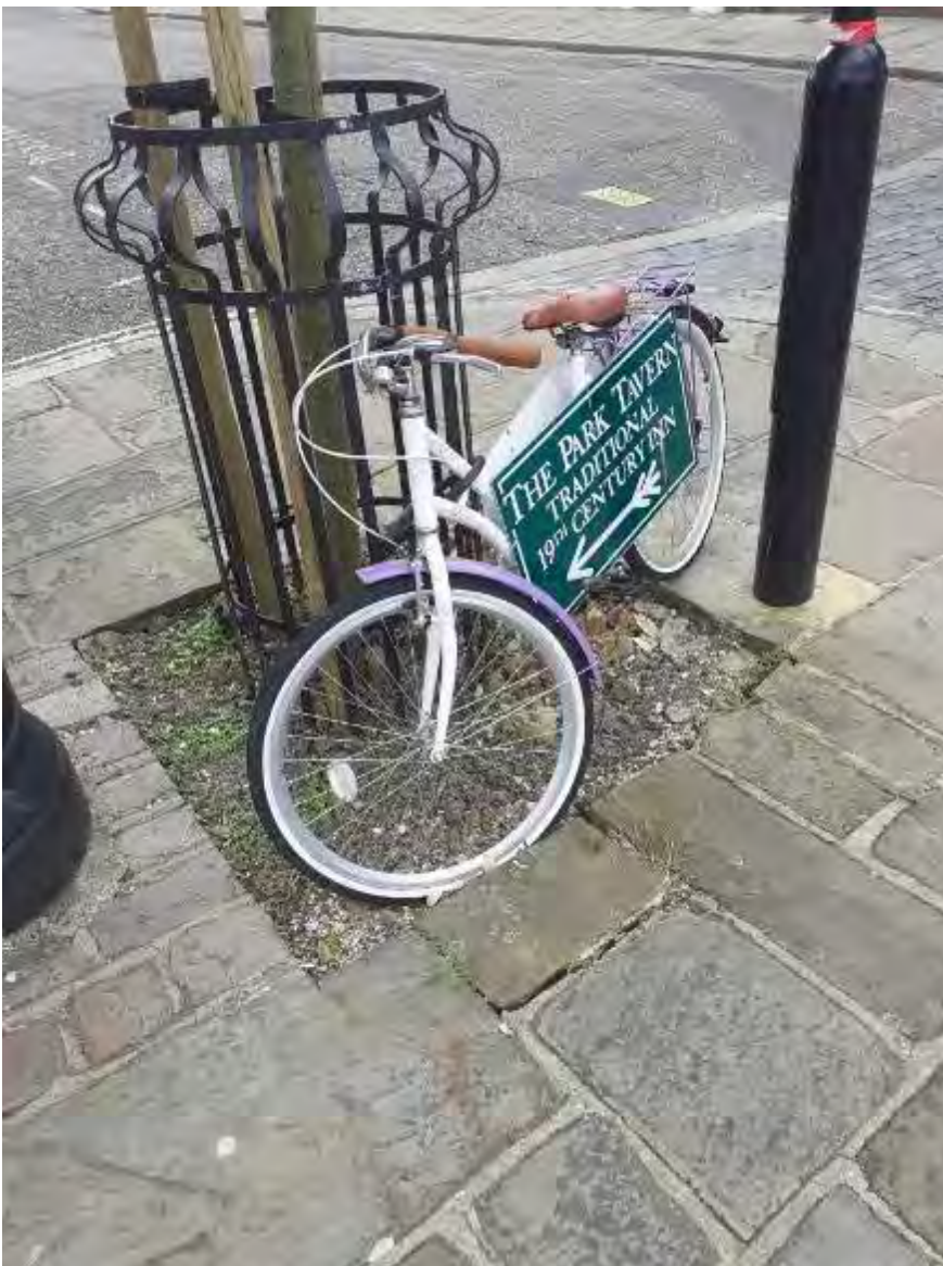
Lack of proper edgings or tree pit protection. Inappropriate street clutter / advertising
