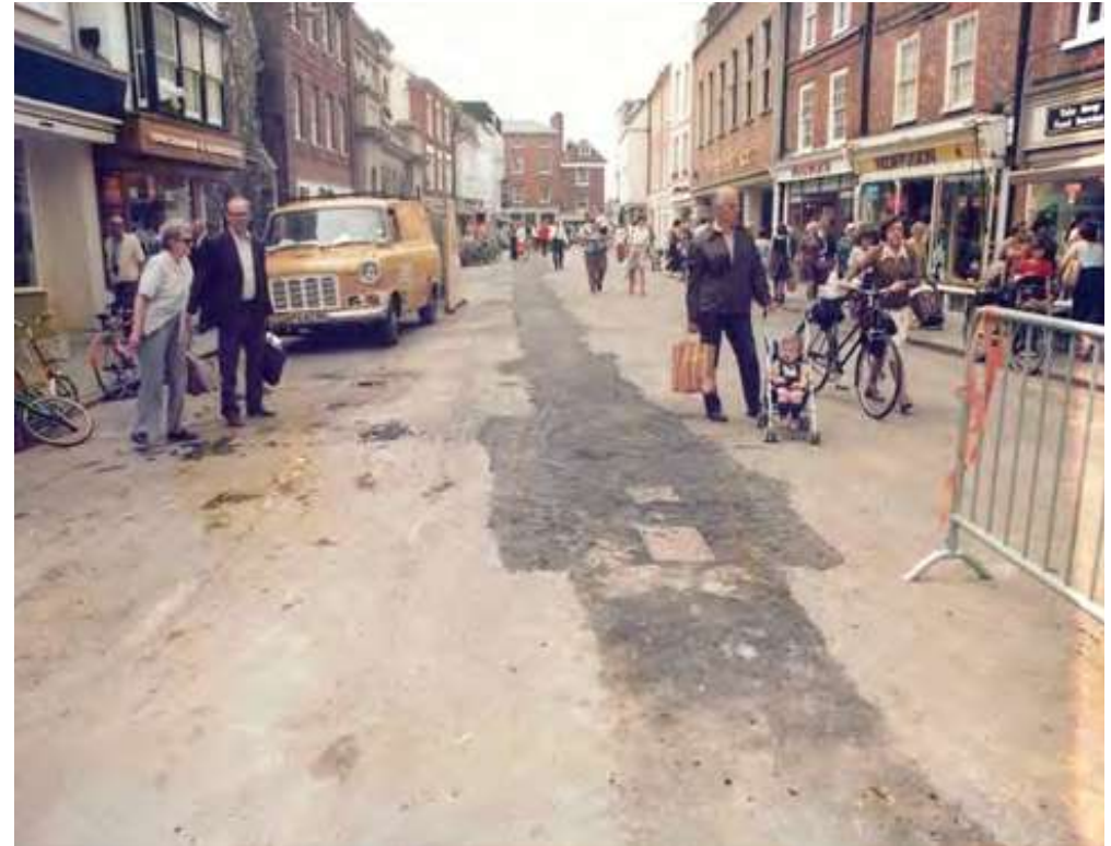
Figure 2.3 North Street looking towards Chichester Cross (just out of shot) circa 1970's, this photo would suggest that the road had been closed and works to the paving were shortly beginning, the camber on the road and position of existing kerbs and footways can be seen, bicycles can be seen in the distance (left-hand side behind the van) parked on the road.
