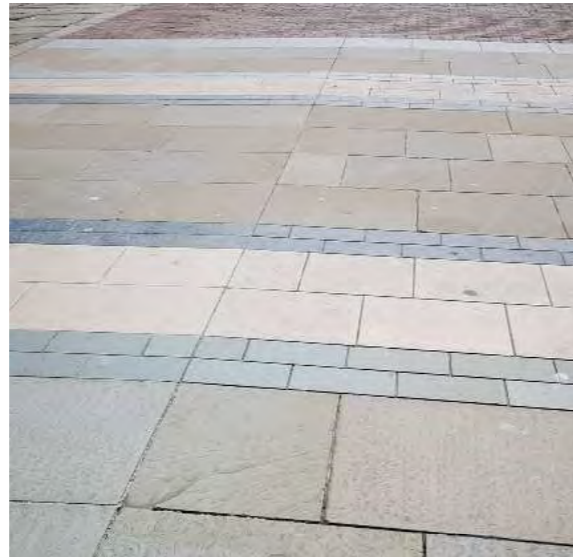
Trial panel on North St
