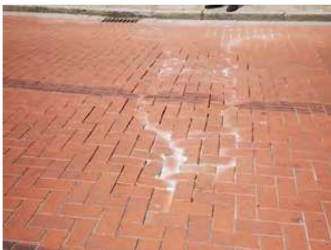
Figure 6.4: Block paving irregularities
