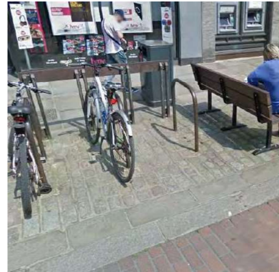
Tumbled light grey granite setts to furniture areas on North St & East St
