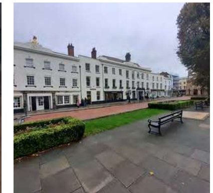
Concrete slabs around the cathedral grounds
