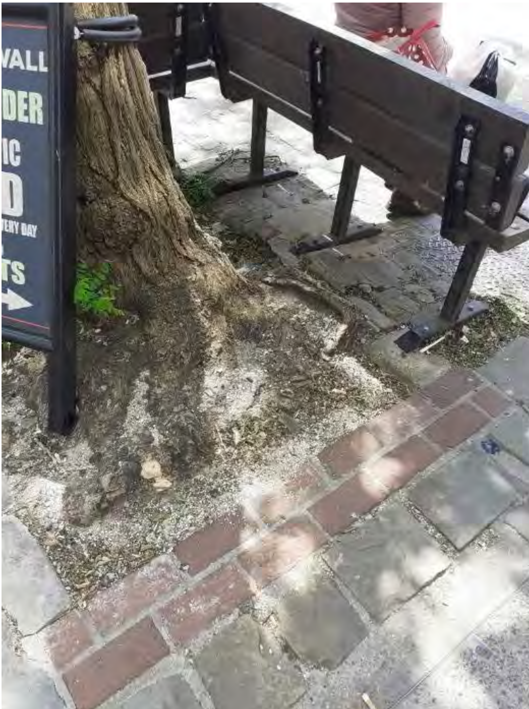
Tree health likely to suffer, eclectic use of materials. Tree roots pulling up paving due to insufficient rooting volume and medium. Lot of clutter. It would be good to understand how these trees were planted and scope for improving the rooting medium.
