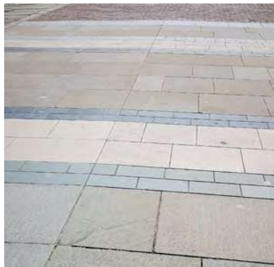
Trial panel on North St
