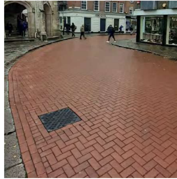
Red clay paviours laid herringbone to bus route
