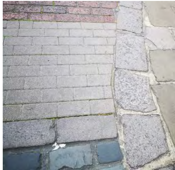
Buff paviours to gateways to pedestrian zones
