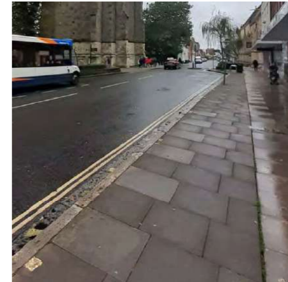
Concrete slabs & asphalt to West Street
