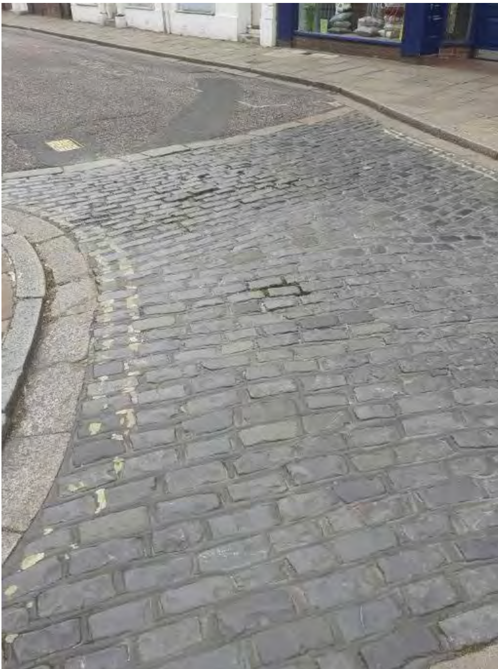
Mortar joints / grouting beginning to fail. Yellow lines ineffective (and inappropriate, perhaps use zonal restrictions) Kerbs and channel failing.
