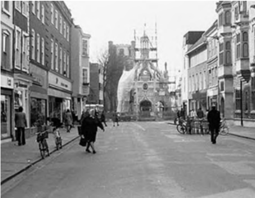
Figure 2.2 East Street looking towards the Chichester Cross, circa late 1960's / early 1970's, note camber of road and the position of existing kerbs and footways
