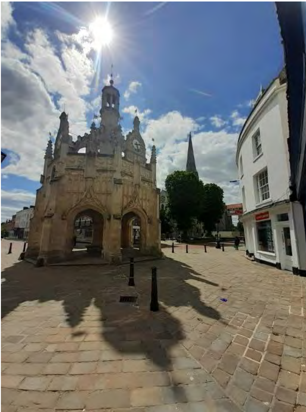
The market cross, this is a key heritage asset. Radiating Octagonal paving causing issues with cuts and maintenance. Contractors clearly struggling to re-lay the stone correctly following repairs.
