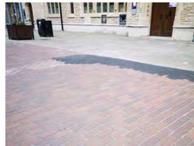
Figure 6.1: Temporary repairs to block paving with asphalt (utilities)
