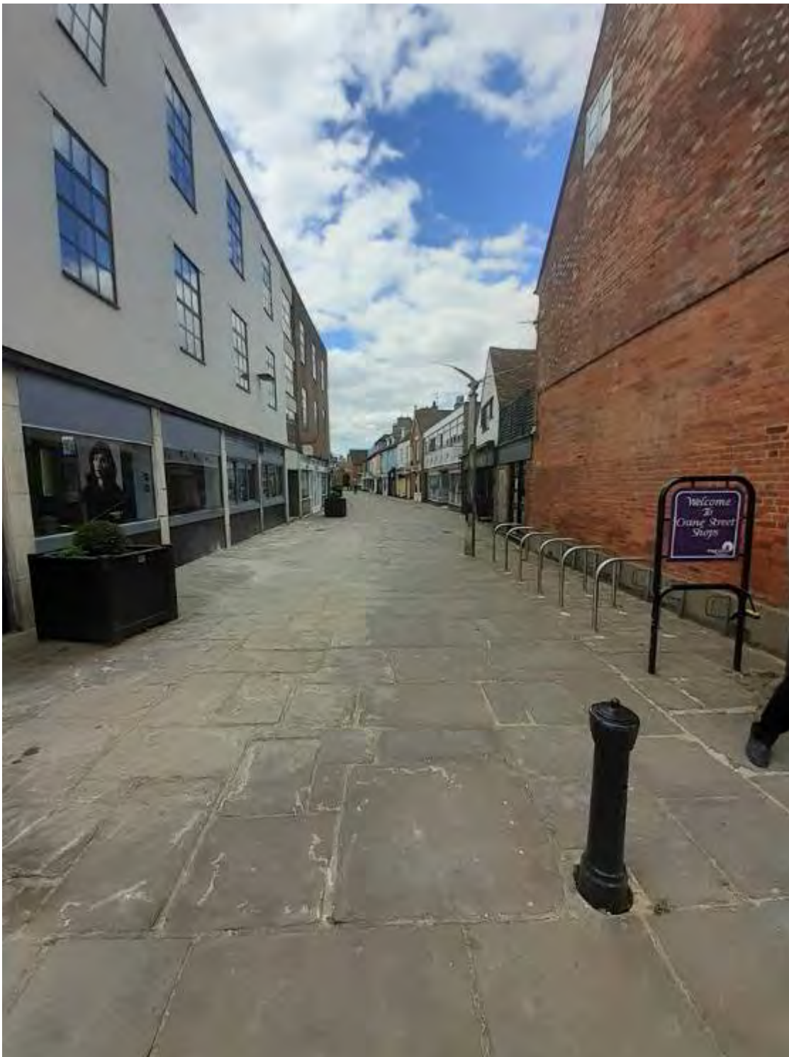
Uninteresting and poor-quality street scene along Crane Street
