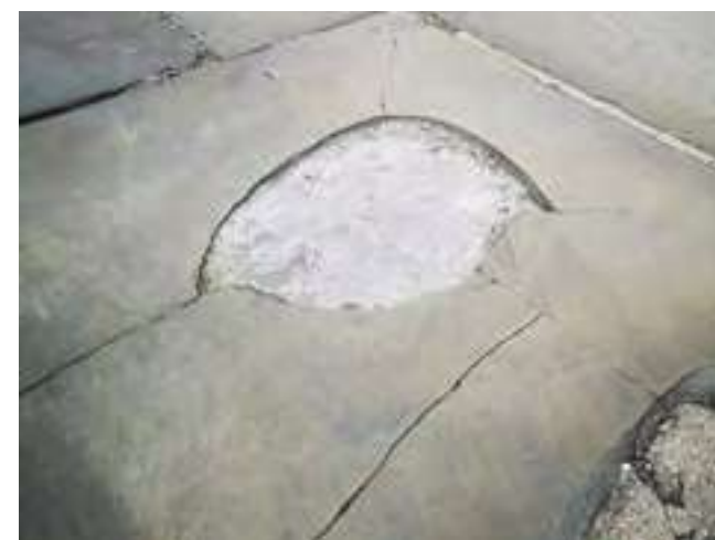
Figure 6.2: Broken slabs repaired with concrete
