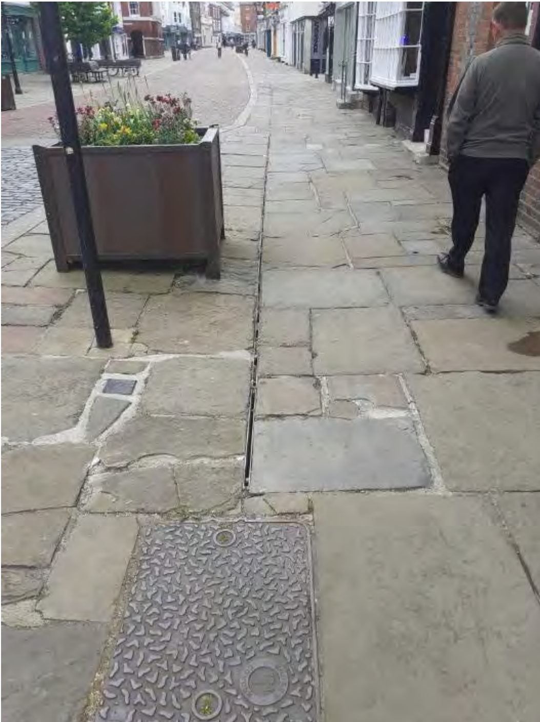
Slot drains blocking up, mortar failing, poor quality colour matching
