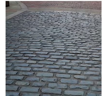
Blue granite setts to gateways to pedestrian zones
