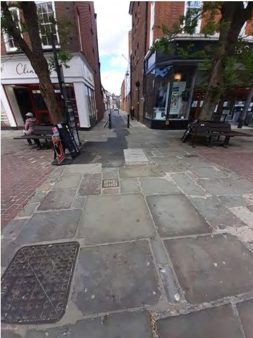
Strange emphasis given to the north south crossroads, when attention and importance should be given to the cross. Need to reconsider hierarchy of materials. Note the extensive tarmac patching.
