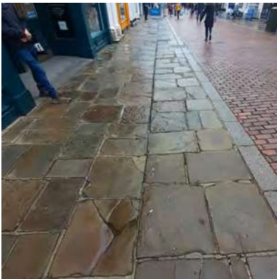
Yorkstone slabs to majority of footways
