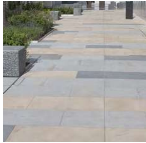
Precedents with Yorkstone paving units
