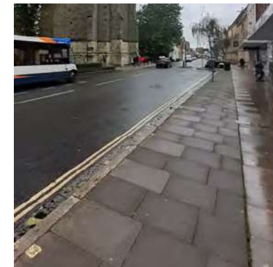
Concrete slabs & asphalt to West Street
