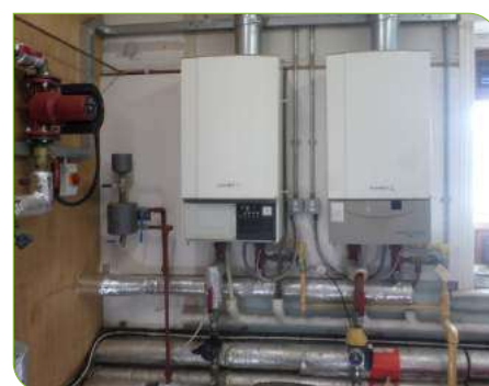
Photo 1 – Main boilers in Council House
