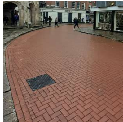
Red pavers laid herringbone to bus route
