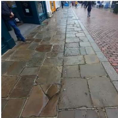
Yorkstone slabs to majority of footways
