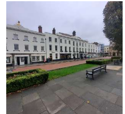
Concrete slabs around the cathedral grounds
