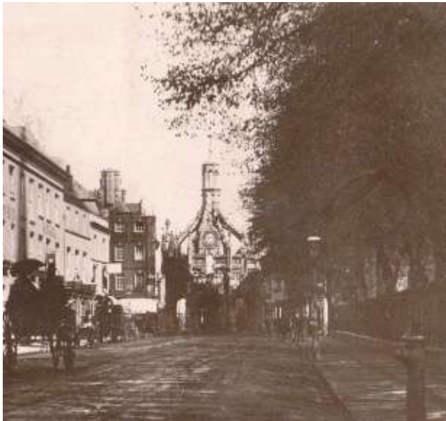
3.3.1 Looking East towards Market Cross (1910) Broad cobbled street with footway & railing to Cathedral ground.
