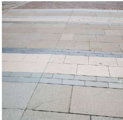
Trial panel on North St
