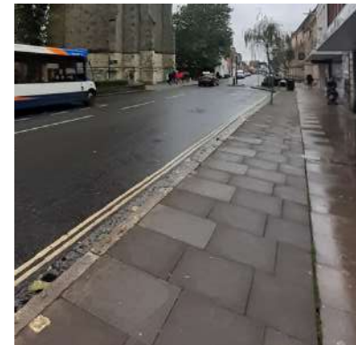
Concrete slabs & asphalt to West Street
