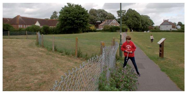
The line of the access path will be retained in most locations to avoid further construction excavation. The path will be resurfaced with a new wearing course and a chip and tar finish. The exception to the position of the path will be the Velyn Avenue entrance where the path will be centralized on the entrance.
