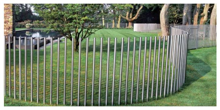
A simple boundary line of steel pins defines the outside foot of the gravel seating bank. This elegant line cannot have invasive footings so will be detailed as free sanding elements.. Density and height of post could vary depending on the intended visual effect and degree of enclosure required.
