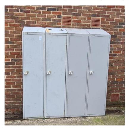
The original lockers were installed in 2022 supplied by CDC and we assisted in fitting them. The issue with the lockers are they are only internal grade lockers and therefore they have rusted, let in water, locks seize and people then get frustrated and break into them.
