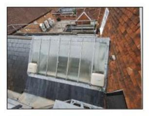
IMAGE 1 VIEW OF THE EXISTING ROOF LANTERN FROM THE NORTH SHOWING EXISTING MECHANICAL VENTS.
