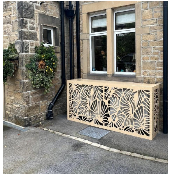
Air source heat pumps can be enclosed to suit the context .
