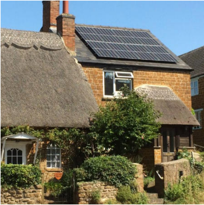
Solar panels can be sensitively located on appropriate roof slopes
