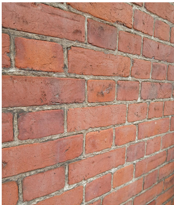
Georgian brick work burnt headers chichester .
