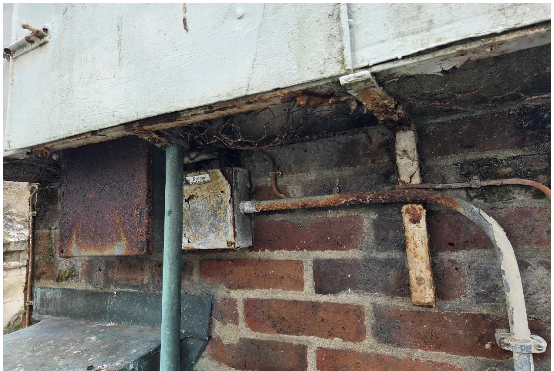
59. This photo shows the corrosion to the support brackets beneath the clock casing.
