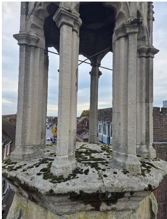
56. The piers are heavily eroded and there is much moss cover on the base.
