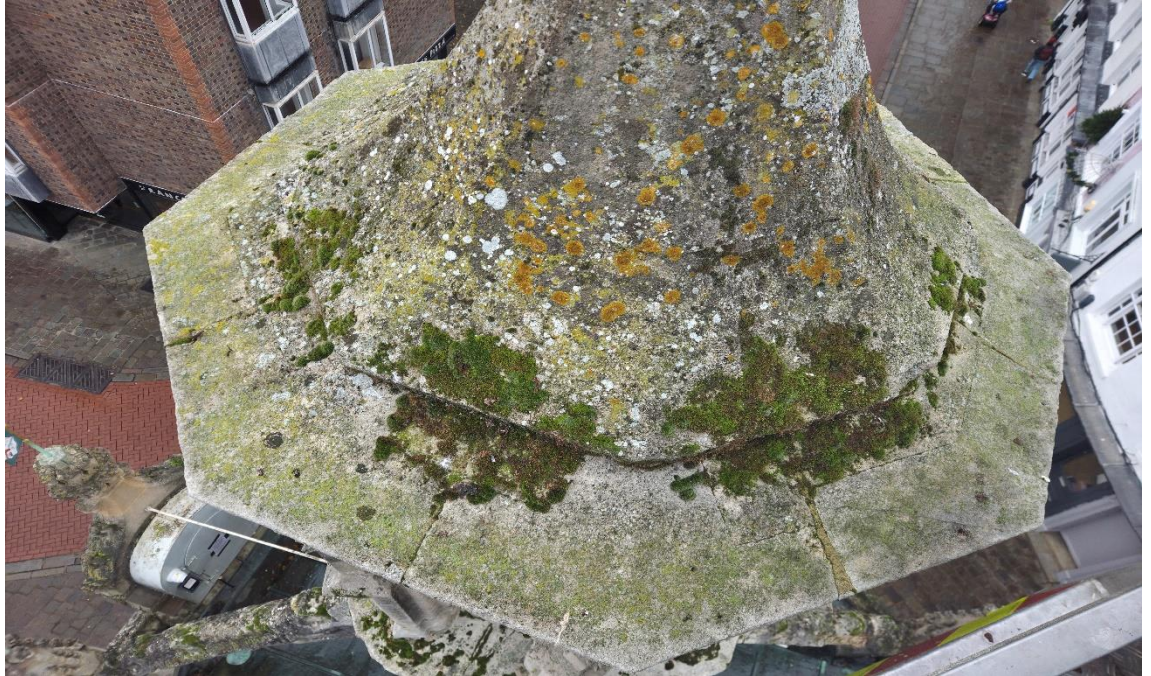
56. The piers are heavily eroded and there is much moss cover on the base.
